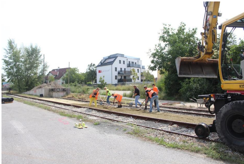
Figure 1. Installation of geotextiles in Vienna Breitenlee (Wiegele)
